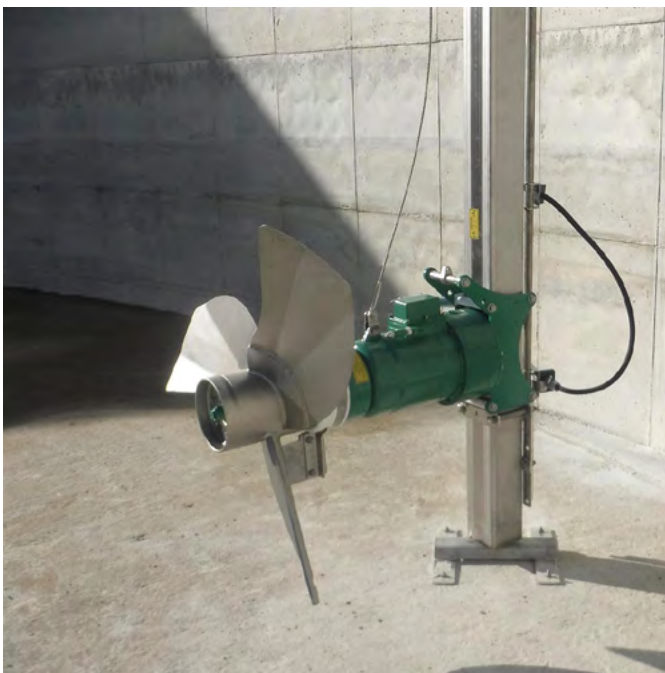
4G with EV - Closed tank
