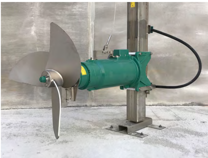
3G - Concrete tank
