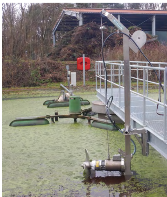
2A with EV - Open tank
