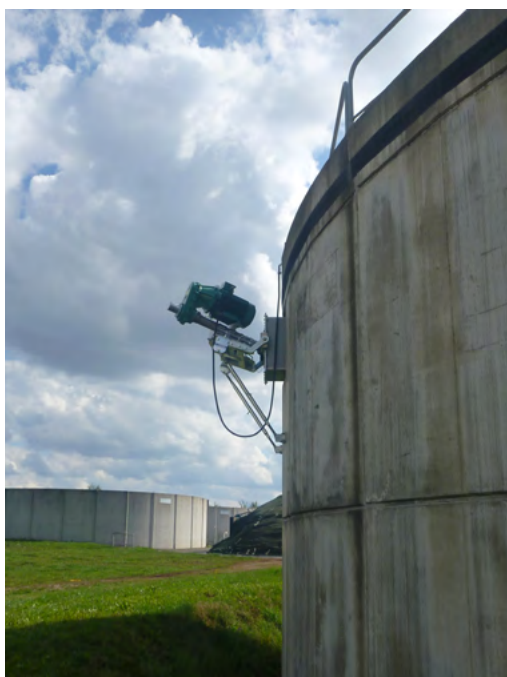
FR SP - Concrete tank
