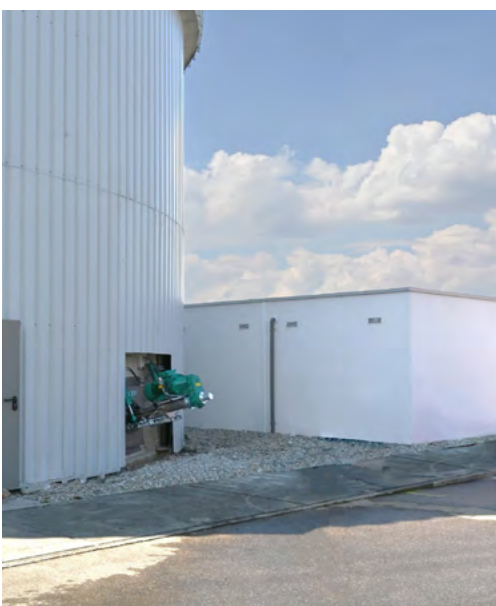
FT - Closed tank
