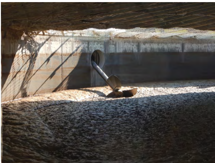
FTX - Concrete tank
